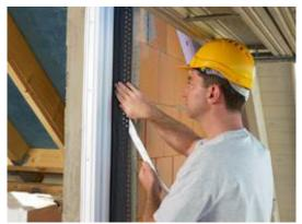
The black coloured, single-sided high-performance adhesive tape Fentrim 2 is the optimal solution for permanent windtight and driving-rain proof bonding of window and door frames in **solid construction on the outside**. It is therefore perfectly suited to many commercial and residential applications where solid structure facades are specified. A perforated edge zone provides perfect keying in for final coating like render, acratex or similar trowelled finishes.
